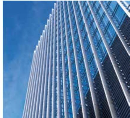
▲ Tall office building. Sleek, vertically mounted CS Airfoil® blades are the centrepiece of this unique and daring piece of architecture, providing effective shading due to the south-east orientation of the building
