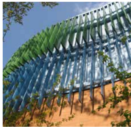
▲ Museum. Colourful CS Airfoil® blades with our high quality powder coated finish follow the silhouette of the building creating an artful effect of an otherwise unappealing façade.
